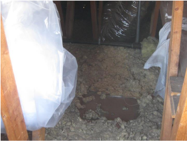
Picture 13: Attic Insulation
