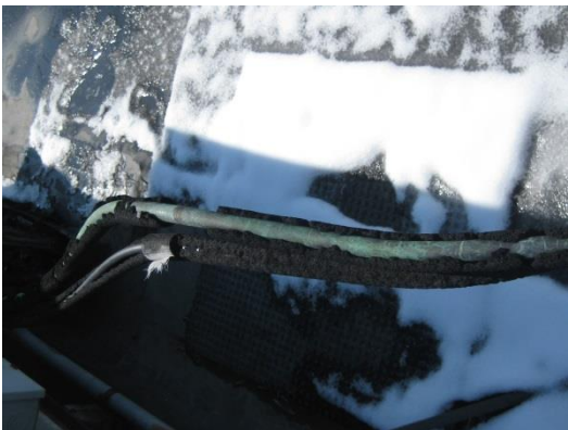
Picture 12: Damaged Suction Line Insulation
