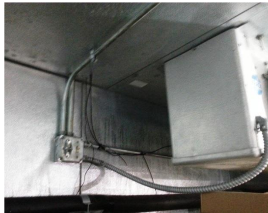
Photo 12: No Icing Post-Retrofit
