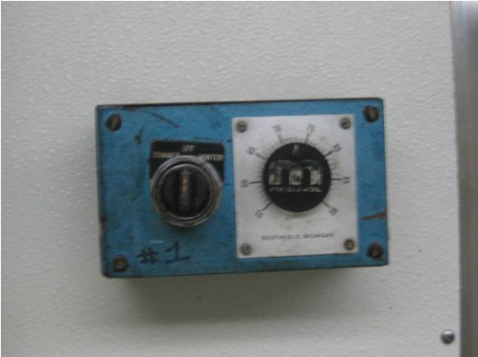
Picture 11: Temperature Control for Make-up Air
