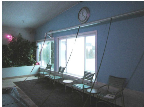
FIGURE 1: SOLID POOL COVER AND PULLEY SYSTEM USED TO RETRACT POOL COVER
