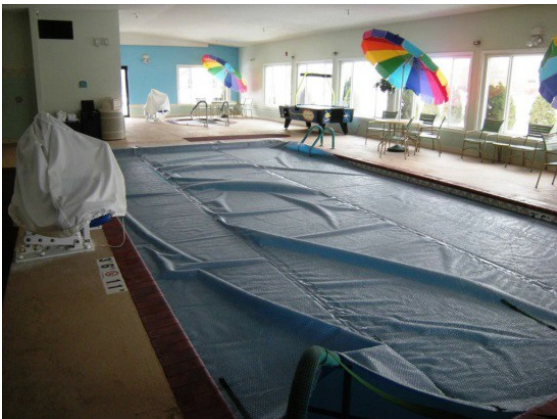
FIGURE 1: SOLID POOL COVER AND PULLEY SYSTEM USED TO RETRACT POOL COVER
