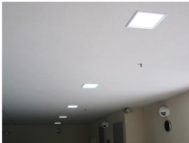
FIGURE 8: POOL AREA LIGHTING
