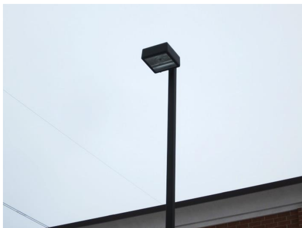
FIGURE 5: PARKING LOT POLE FIXTURE
