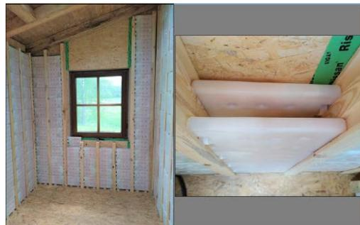
FIGURE 12 PCM INSTALLATION
