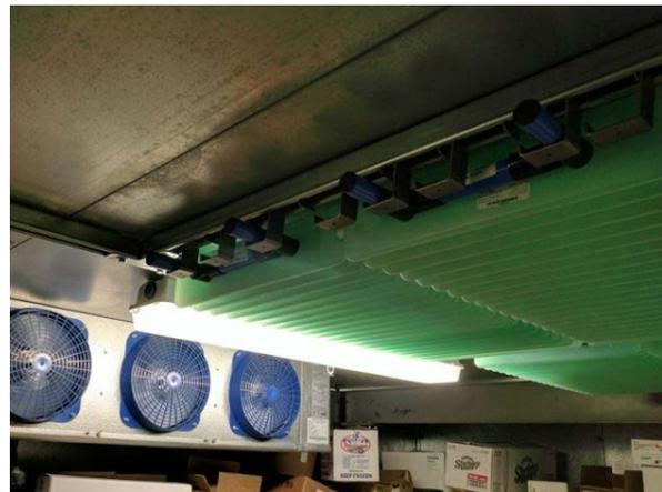
FIGURE 6 SALT-WATER PCM APPLICATION[7]
