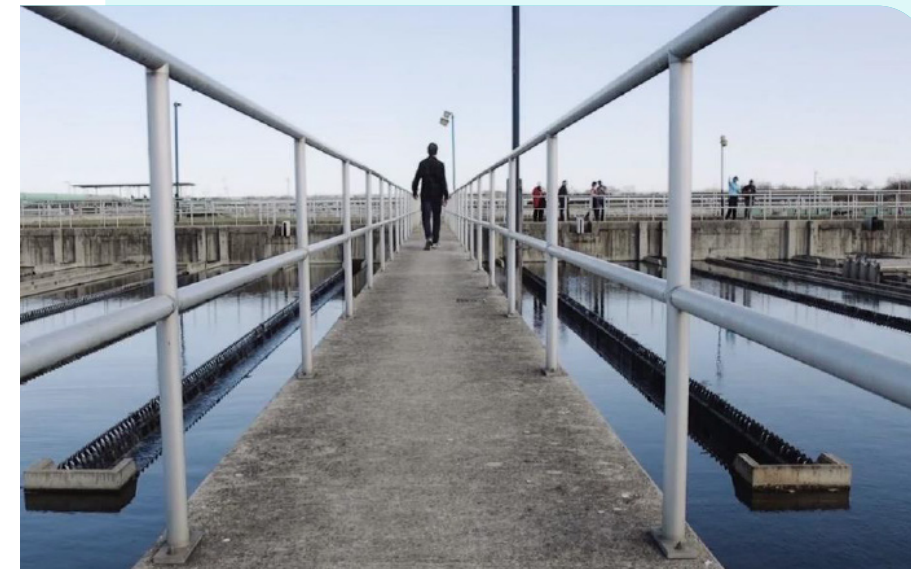
Optimizing water and wastewater treatment is one technical subject of SAWS' energy management strategy. Staff training on energy issues is building capacity for the future. (Photo courtesy of SAWS)
