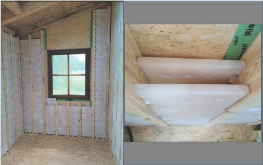
Figure 12. PCM Installation
