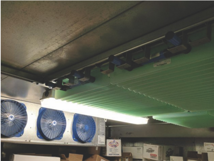
Figure 6. Salt-water PCM Application (Source: Viking Cold Solutions)
